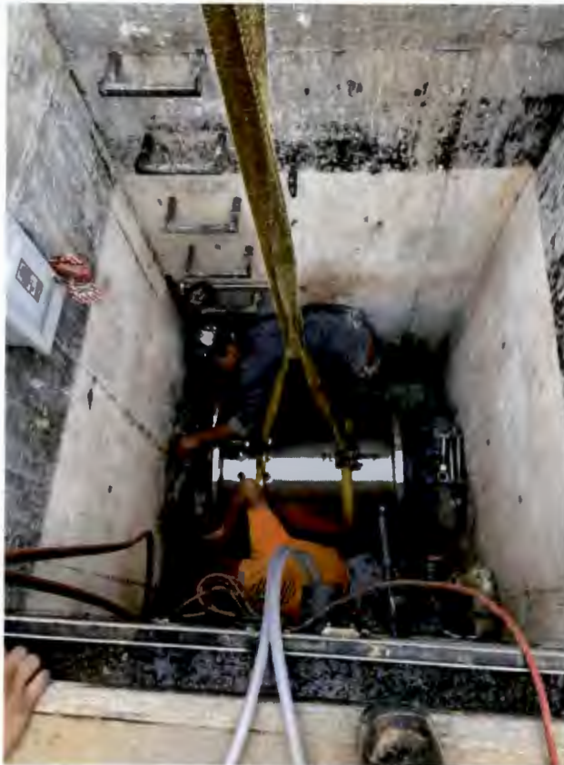
Static Post Mixer Installation (October 2022)
