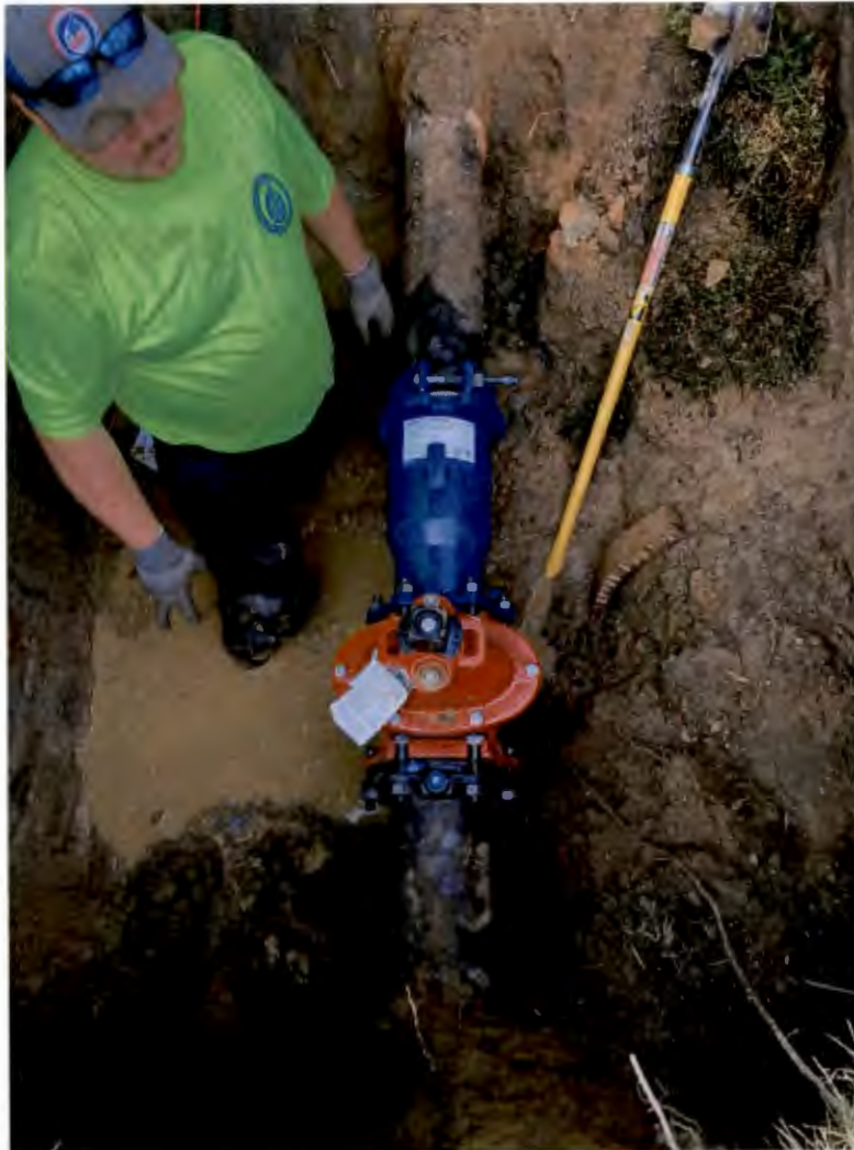
New Mainline Valve Installation at Terrace Acres Drive/Terrace Acres Circle Intersection (September 2022)
