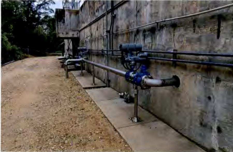
Basin 3 Sludge Waste Piping (October 2022)
